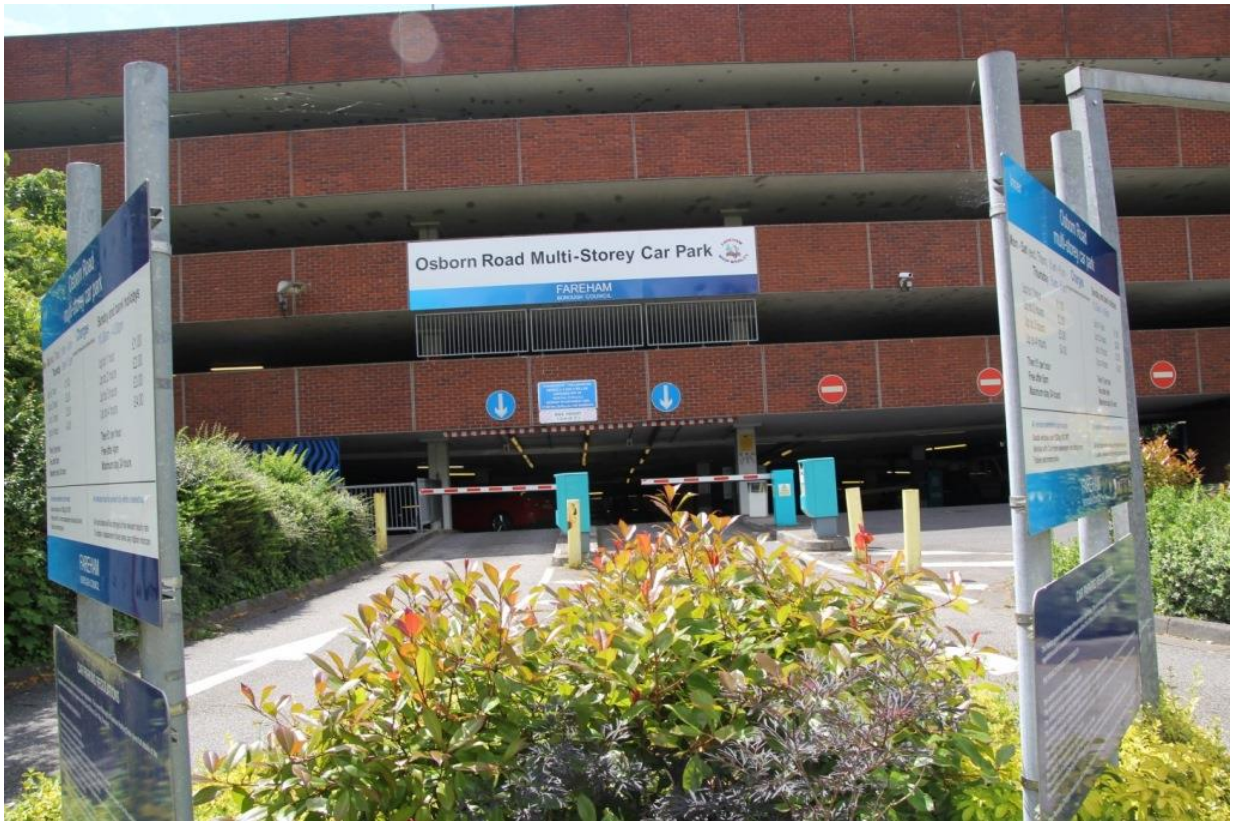
Osborn Road Multi-Story Car Park
